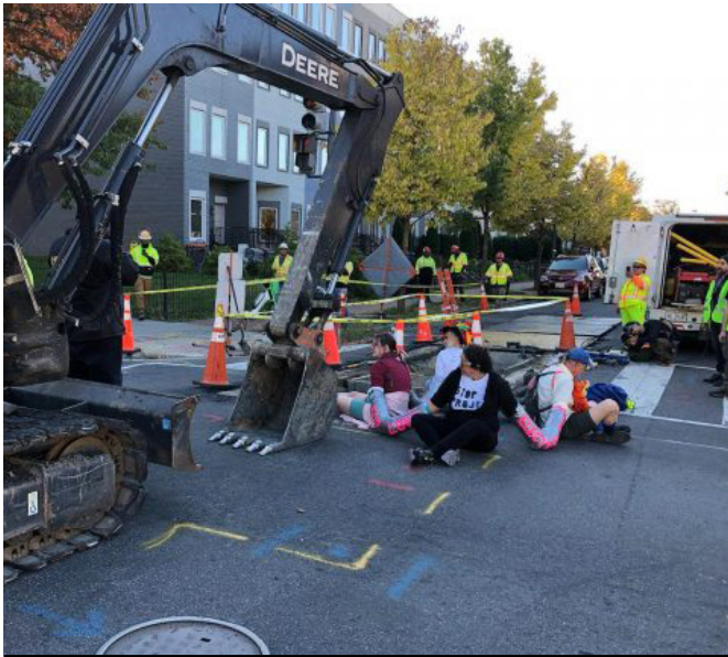
Activists stopped work on Washington Gas' Project Pipes by locking themselves together over the construction site. They were eventually removed by police and arrested. Over 50 protesters joined in the action chanting, playing music, waving banners, and supporting their locked down friends. | Photo by Miles Amore
